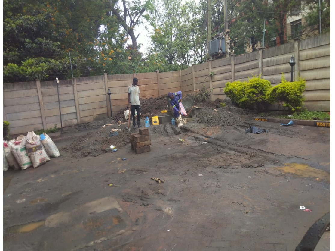
Ongoing borehole drilling
